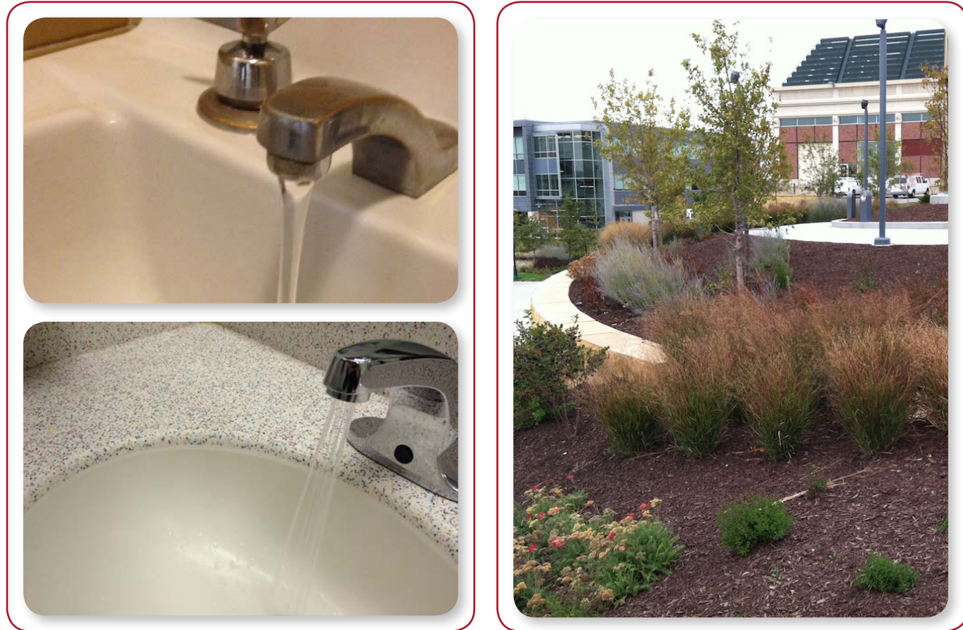
Figure 14 Low-Flow Faucet Aerators. The faucet shown on top has no aerator installed. Faucet aerators introduce tiny air bubbles into the stream to reduce the flow and reduce splashing. Low-flow faucet aerators, shown at bottom, go even further to reduce the flow. Use of aerators is not consistent throughout UNMC/NM's buildings, but they could reduce faucet water use by 30 percent or more.
